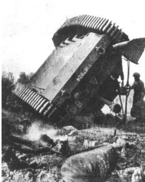
Overturned “Cromwell” tank which leaped in the air due to a close bomb explosion during the friendly fire (Source: Regimental History of the 10 th Mounted Rifles Regiment, Nuremberg 1947)
